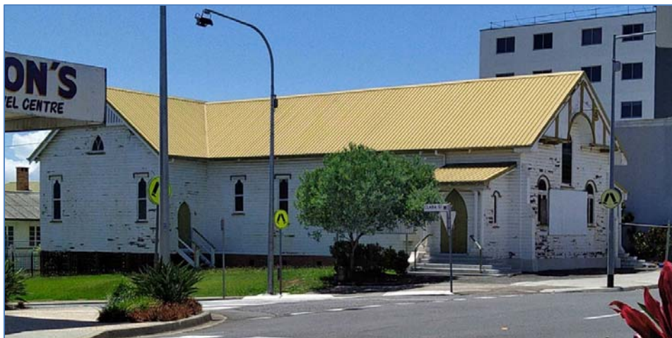
Former Wynnum Baptist Church in a dilapidated state (2021) (Photo: D Parker)
